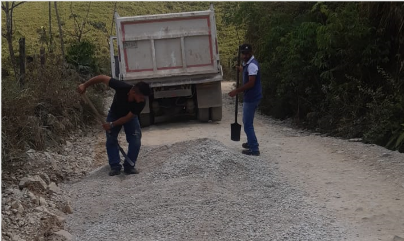
Restoration work on the road to La Danta, Calidra Colombia.
